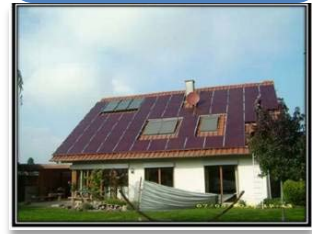
Residential Rooftop PV system
